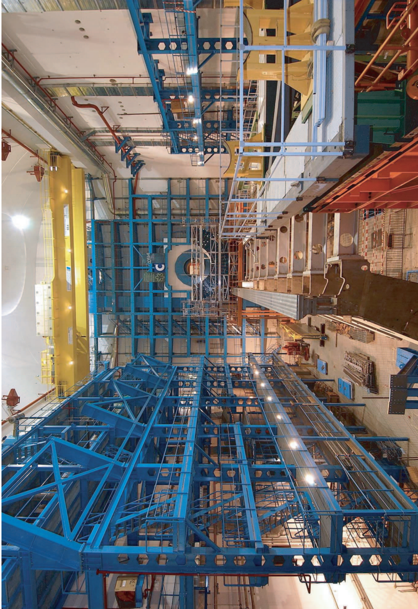
Figure C.2: The ATLAS cavern as in September 2004. The first detector parts, the TileCal has been lowered and are being completed. In the front, rails can be seen for the horizontal movement of detector parts.
