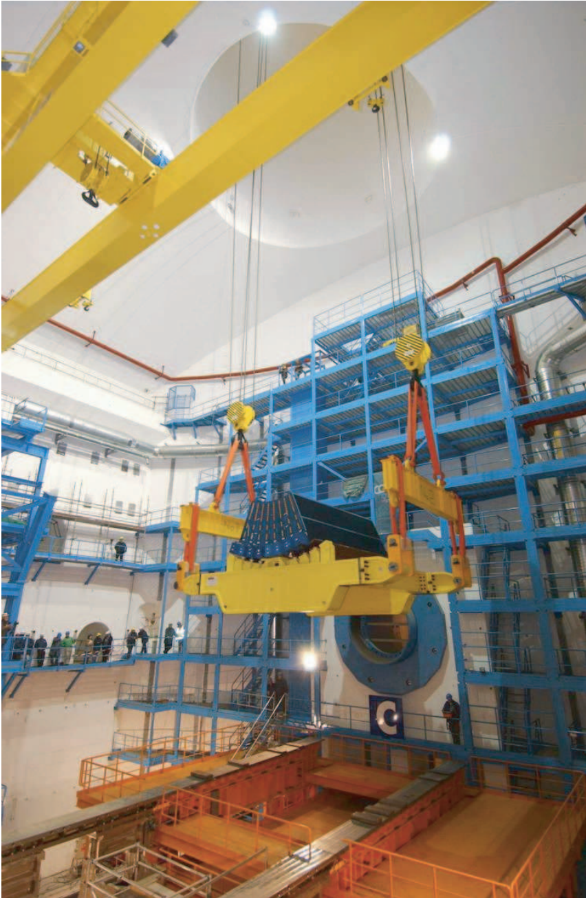
Figure C.3: Tile Calorimeter being lowered into the ATLAS Cavern. The TileCal will be completed in the Cavern into a cylinder.
