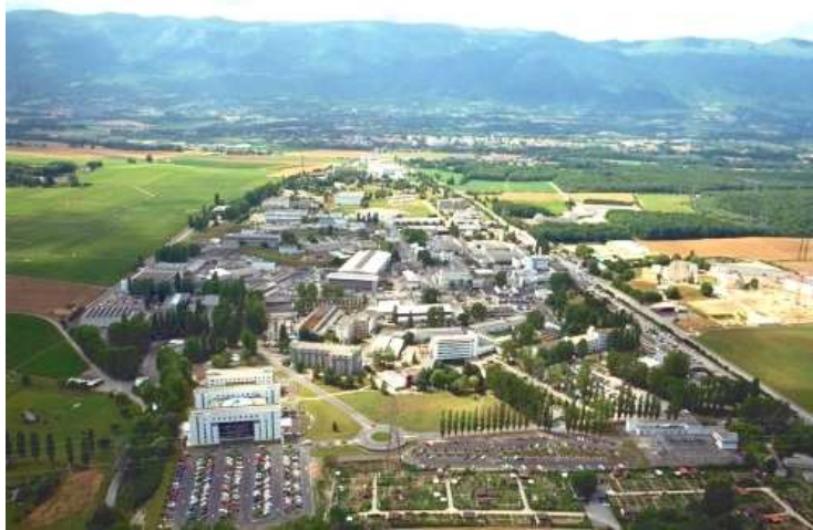
Figure 2.2: CERN seen from the air. The large white building in front-left is the ATLAS building. In the background are the Jura mountains.
